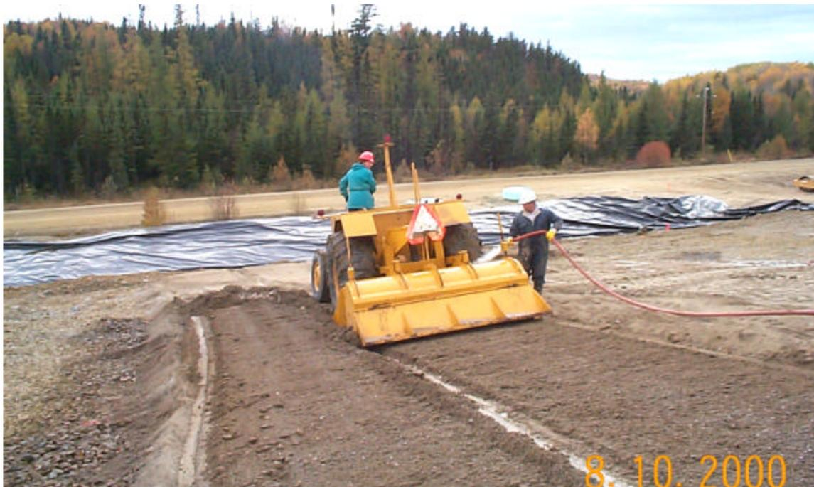
Figure 5. Moisture conditioning and mixing the first lift of the sand-bentonite mixture barrier layer (from OKC 2001).
