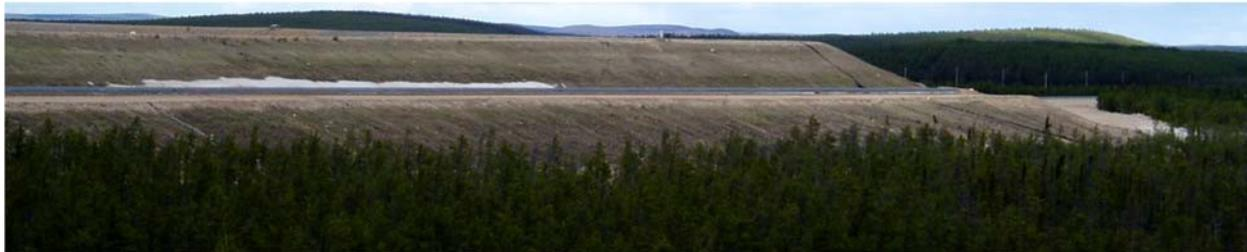
The current AGTMF landform features planar, linear side slopes rising 20 m above the surrounding landscape. Unfortunately, for reasons of long-term geotechnical stability and physical containment of tailings, it was not possible to substantially change the current shape of the perimeter embankments. Nonetheless, the following design concepts were identified to improve the aesthetics of the final landform:
