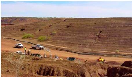
**The greatest physical risks to reclaimed landscapes are gully erosion and failure of surface water drainage courses.**
